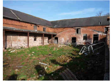
Unit No. 4, Unit No. 5 & Unit No. 3
