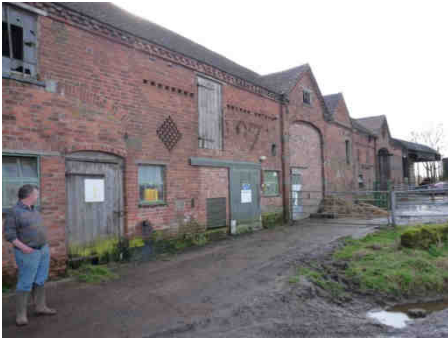
Unit No. 4 Unit No. 5 Unit No. 6
